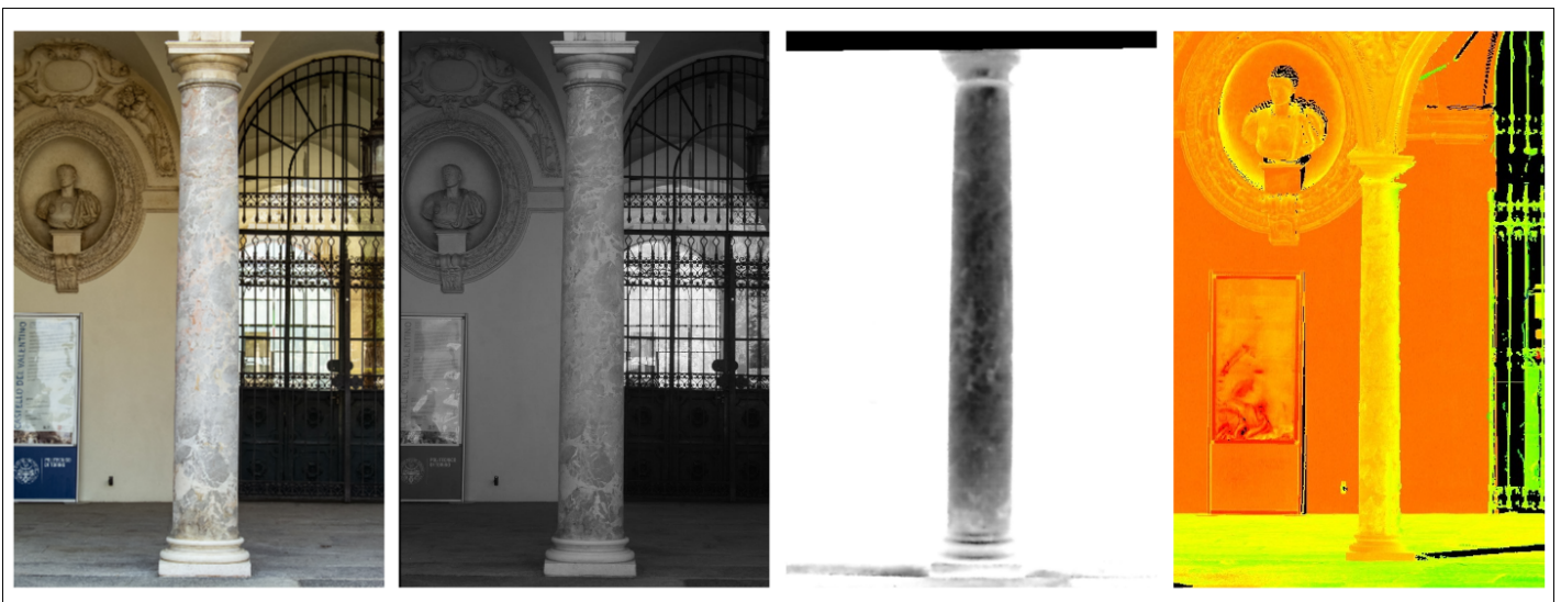
Combination of multisource multidisciplinary results (from left to right): image at the visible spectrum; image at the near infrared spectrum; image at the thermal infrared spectrum; laser scanning-produced point cloud.
